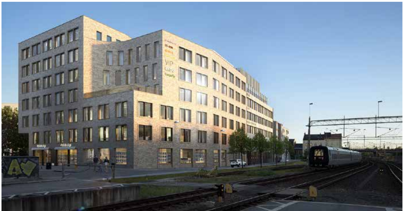
Our new Postterminalen project is centrally located in Lund, adjacent to Lund's central station and neighbouring the municipal office building Kristallen. The 11,000 m 2 office building will be ready to accept tenants in spring 2018.
