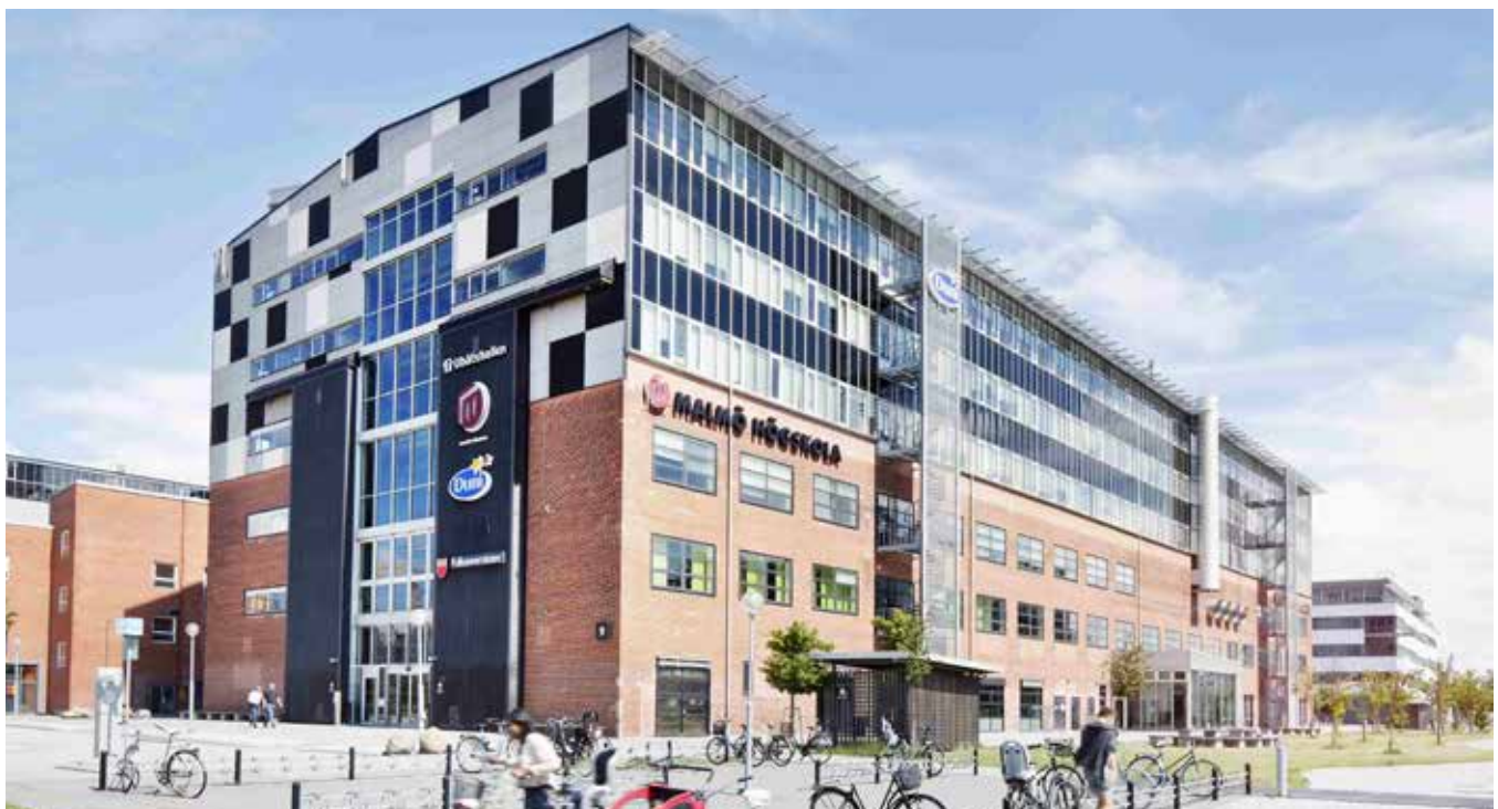
The Ubåtshallen property in Dockan is being rebuilt for Försäkringskassan (the Swedish Social Insurance Agency), which has signed a lease for 12,300 m 2 . For a number of years, both Malmö University and Mediegymsnaset held courses at this address. The first five floors of the building will now be converted to dedicated office space. The sixth and top floor is leased by Duni.
