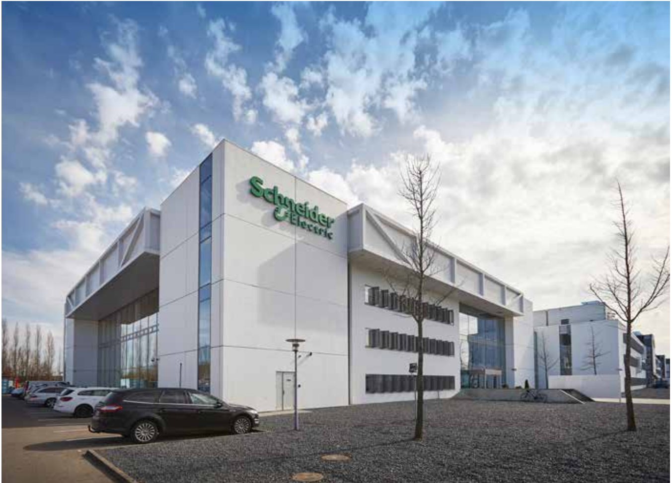
The Lautrupvang 1 property in Ballerup was acquired at the beginning of 2014. Shortly after the acquisition, the entire property was leased to Schneider Electric Denmark and extensive renovation started. One year later, Schneider moved into a modern, efficient and energy-optimised building.
