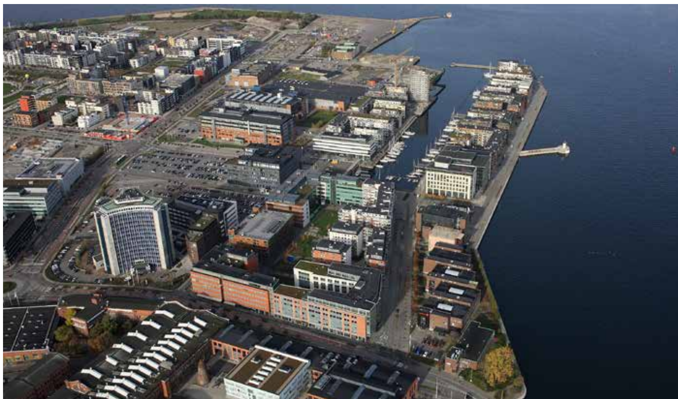
The Dockan development in Malmö remains attractive. SAAB Kockums is leaving Gångtappen but staying in Dockan. The company is moving a few hundred metres to Skrovat 6. Following the renovation, tenants including Länsförsäkringar Skåne are moving into Gångtappen. Orkla Foods has also chosen Wihlborgs in Dockan for the move of its head office from Eslöv to Malmö.
