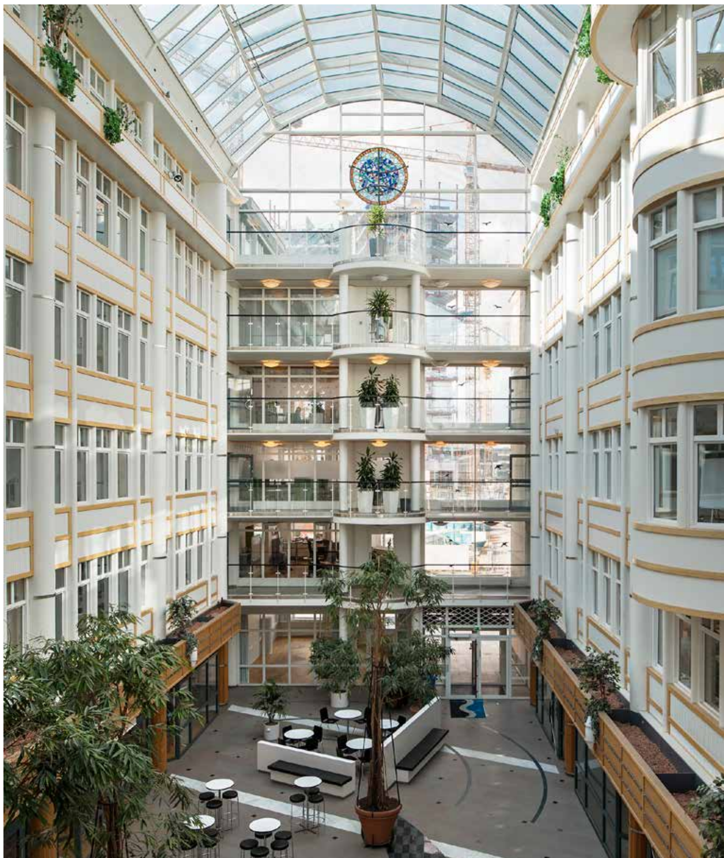
The Våktaren 3 building is located next to one of the entrances to Malmö City Tunnel.
