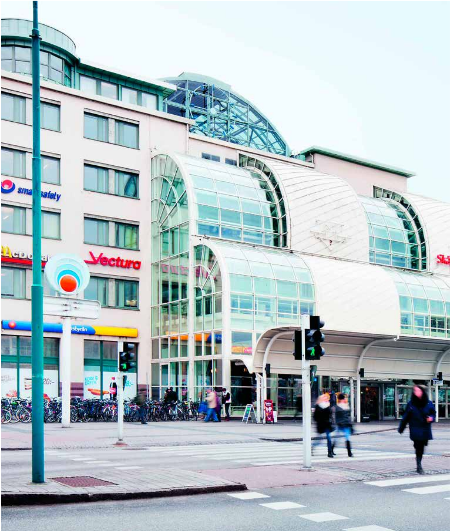
Terminalen 1, Knutpunkten, central Helsingborg. 8,000 m 2 of new office space is being created here. It will be ready for occupancy in spring 2016.
