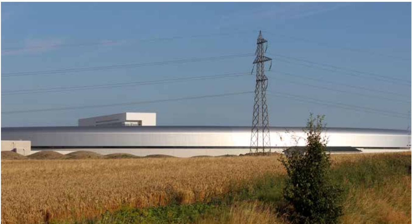
Construction of the MAX IV research centre began in 2010 and is now entering its final phase. In August, the property received MiljöByggnad Gold certification. The facility is scheduled for completion in the second quarter 2015
