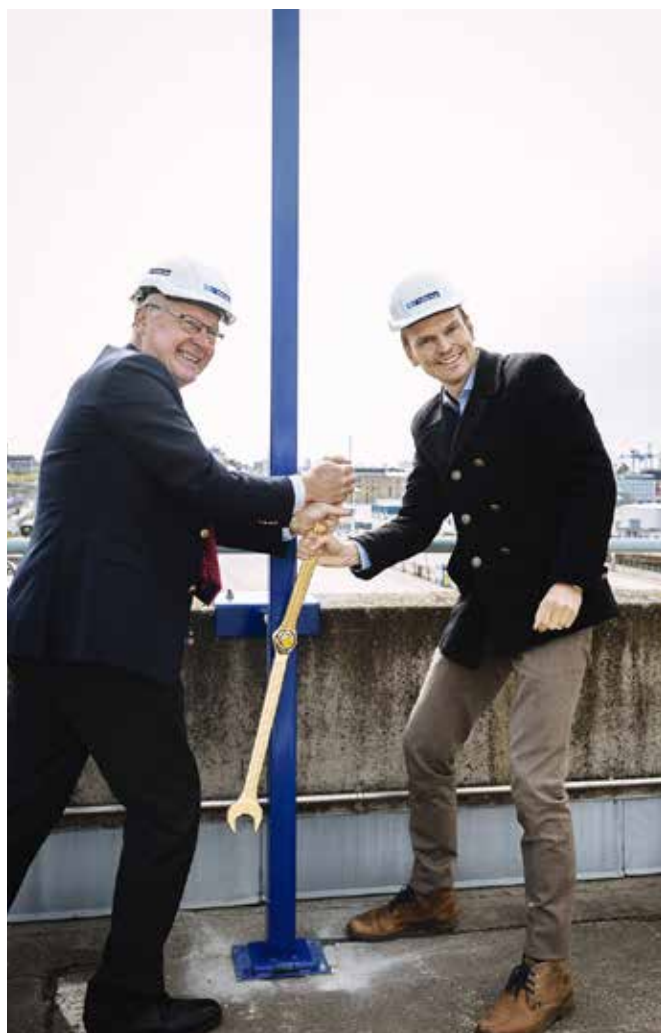
CEO Anders Jarl and Municipal Executive Board Chair Peter Danielsson help to put the roof structure in place for the extension of Knutpunkten, Helsingborg.
