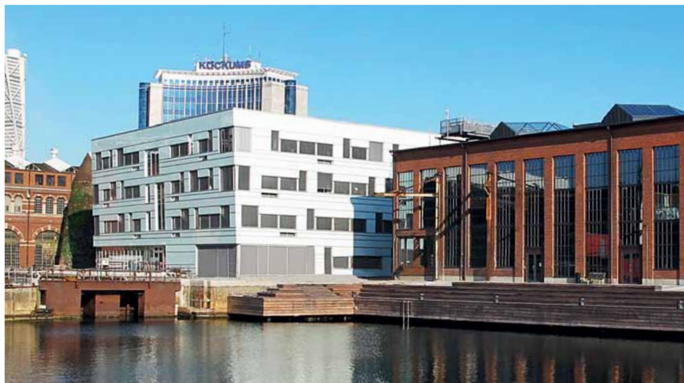
The 2012 Malmö Stadsbyggnadspris (City Architectural Award) went to Media Evolution City, Malmö's new mediacluster. The industrial spirit of the past, dating from Kockums' period of greatness, has been carefully preserved.
