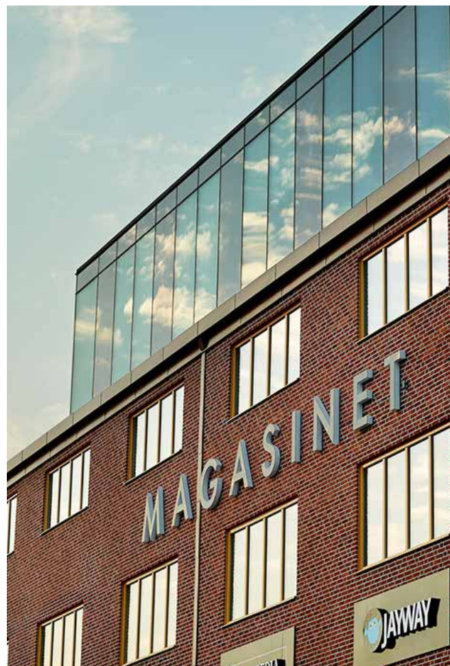
The property Hamnen 22:188, called Magasinet, has been completely renovated.
