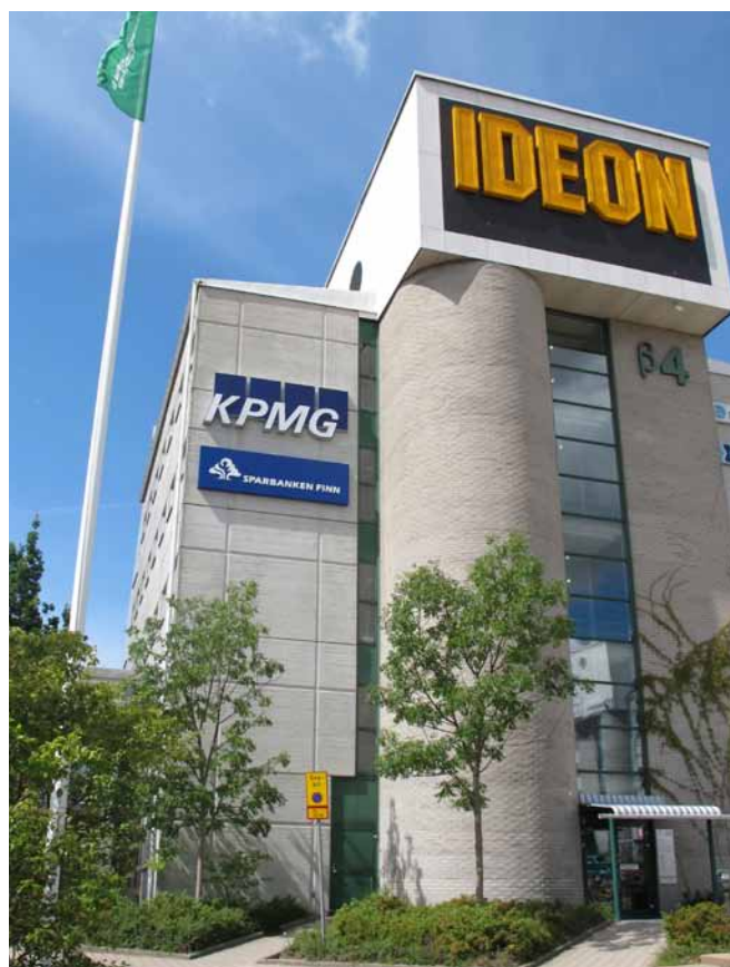
Wihlborgs' office in Lund is situated in the property Vätet 1 at Ideon.
