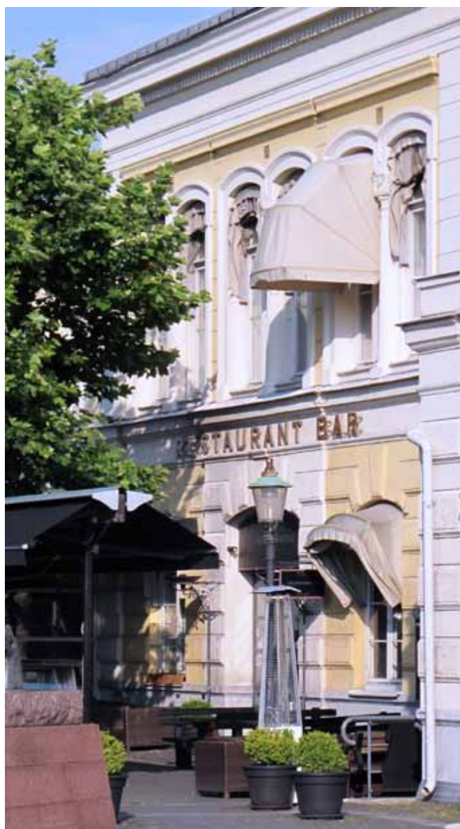
Börshuset in Malmö with its newly renovated facade.
