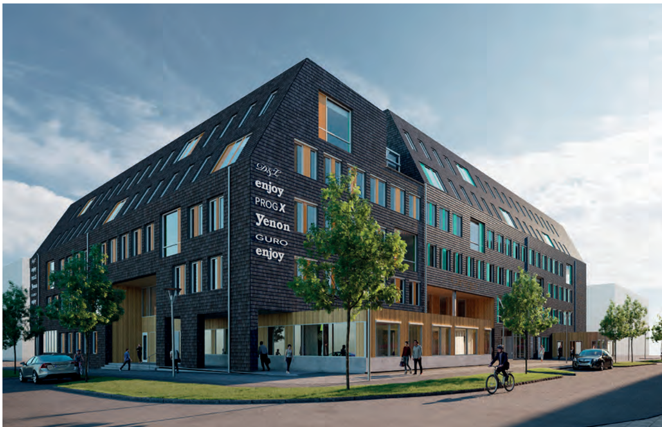
Wihlborgs is constructing the Origo office building in Hyllie with occupancy scheduled for summer 2019. All tenants will have their own balcony and the building includes a shared conference room and bicycle parking facility with showers and changing rooms. The property will be certified to Sweden Green Building Council Gold standard.
