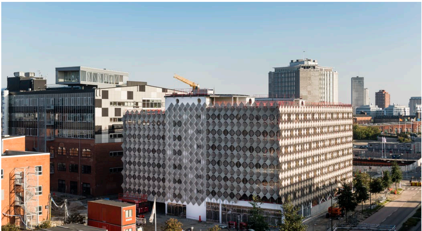
At Wihlborgs' new multistorey car park, Ubåten (Hordaland 1), in Dockan, Malmö, it is possible to recharge your car with solar power.
