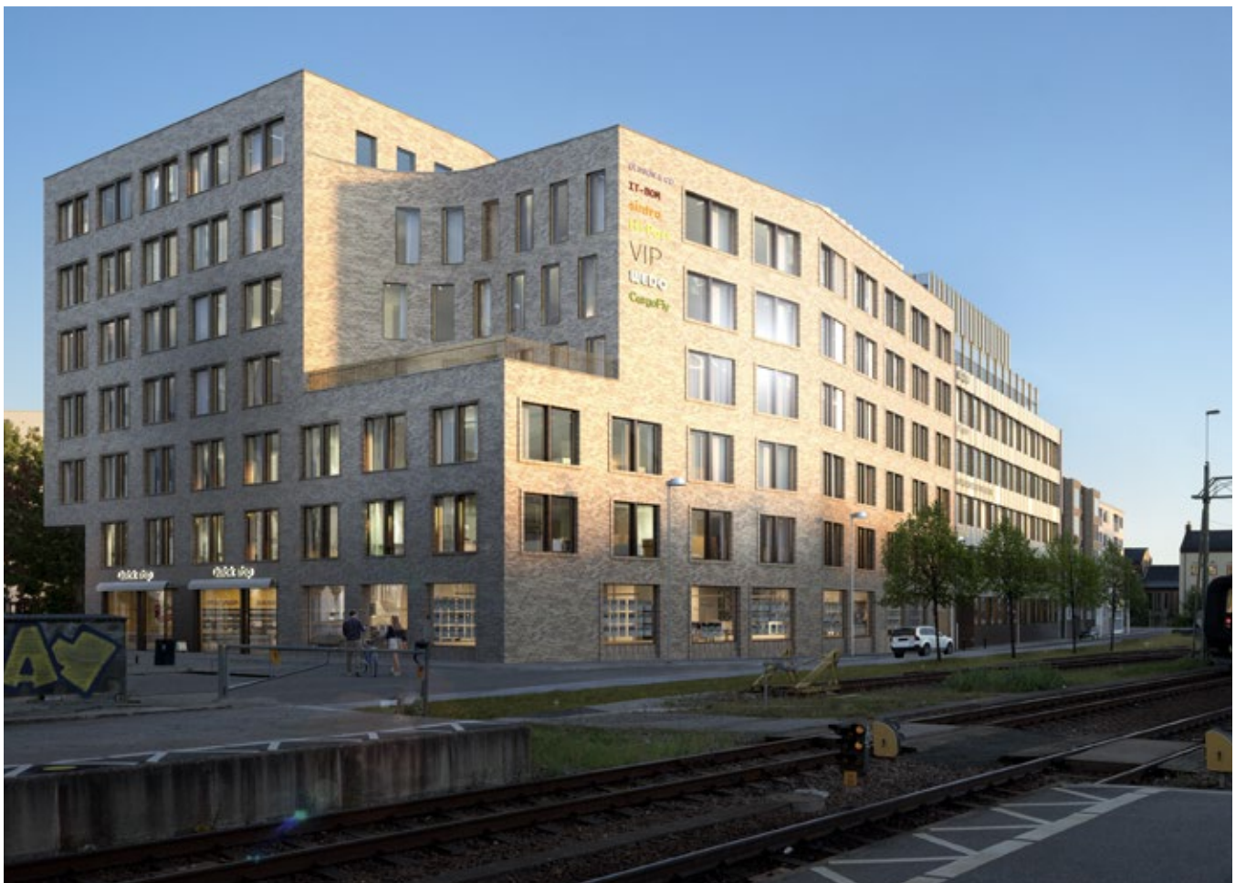
The Posthornet block is being constructed next to Lund Central Station, with occupancy beginning in spring 2018. Folk tandvården Skåne will be one of the tenants, establishing a centre for oral health in the property.
