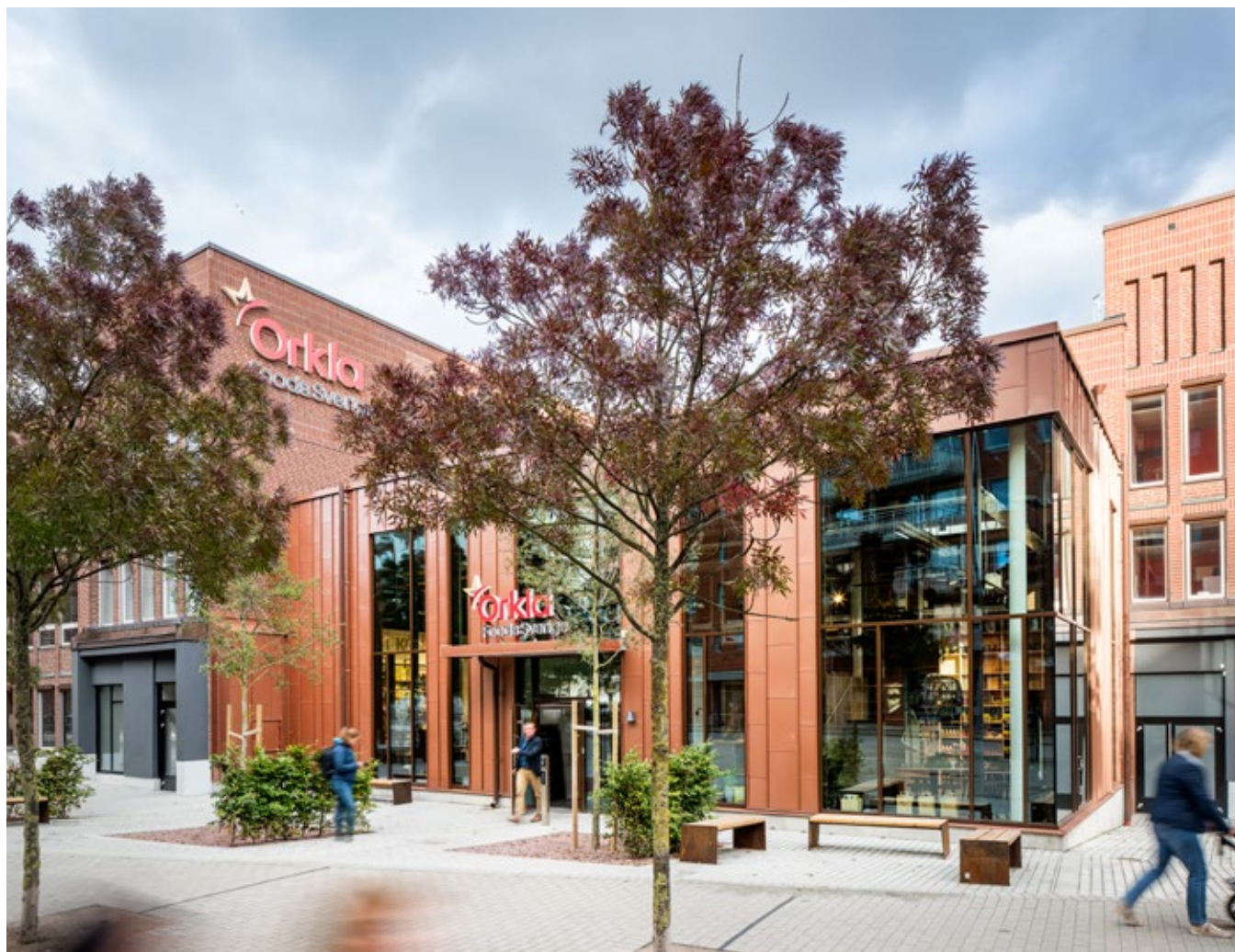
Kranen 1 in Dockan has undergone a major redevelopment and extension for Orkla Foods Sweden who, in spring 2016, moved their headquarters from Eslöv to Malmö.
